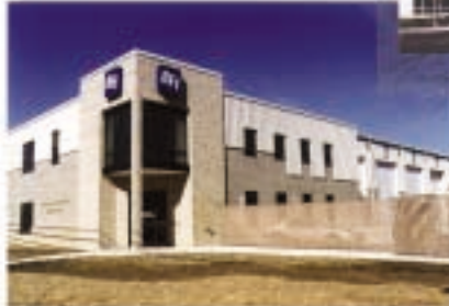
BFI - Office / Maintenance Facility
